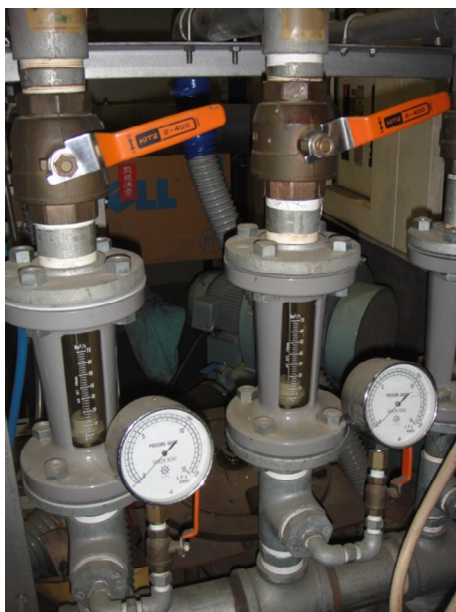
(b) Air rotameters with wide range. (AP-0200 series)
